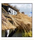
that the roof would take between 4 and 5 tons of wheat straw costing around £1000 per ton. Depending on the climate
